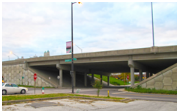
FIGURE 1.5A 16'-7" CLEARANCE ON 3RD STREET UNDER THE HEART OF AMERICA BRIDGE
