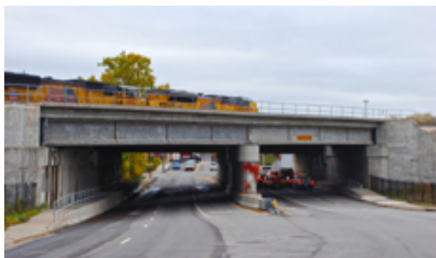
FIGURE 1.5D 14'-8" CLEARANCE ON SOUTHWEST BOULEVARD UNDER THE RAILROAD BRIDGE
