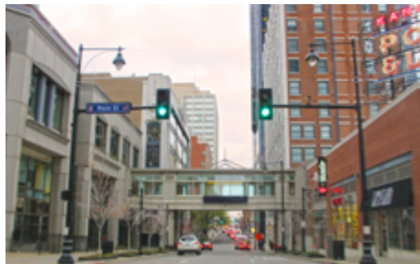
FIGURE 1.5B 15'-10" CLEARANCE ON 12TH STREET NEAR MAIN STREET INTERSECTION
